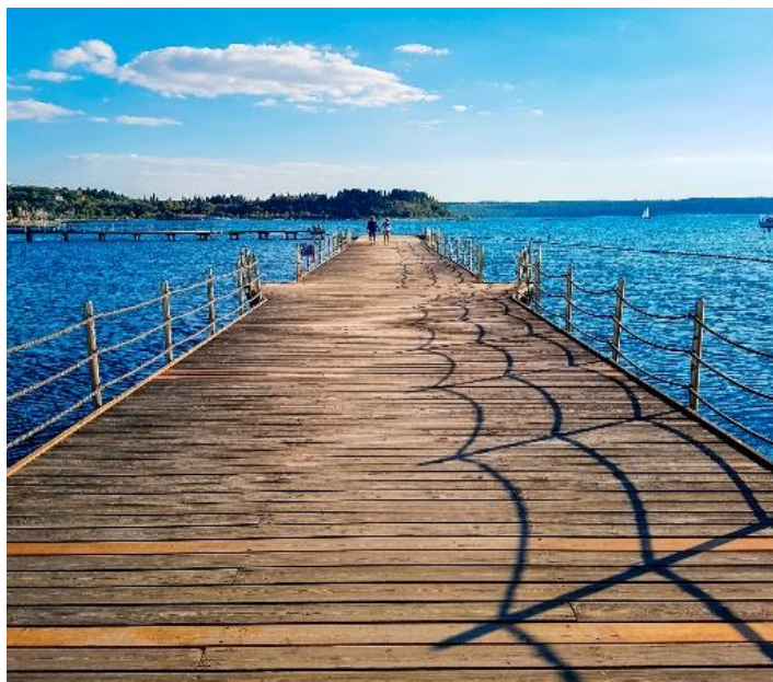
Figure 5. Wood as a part of docks construction (Slovenia360).
