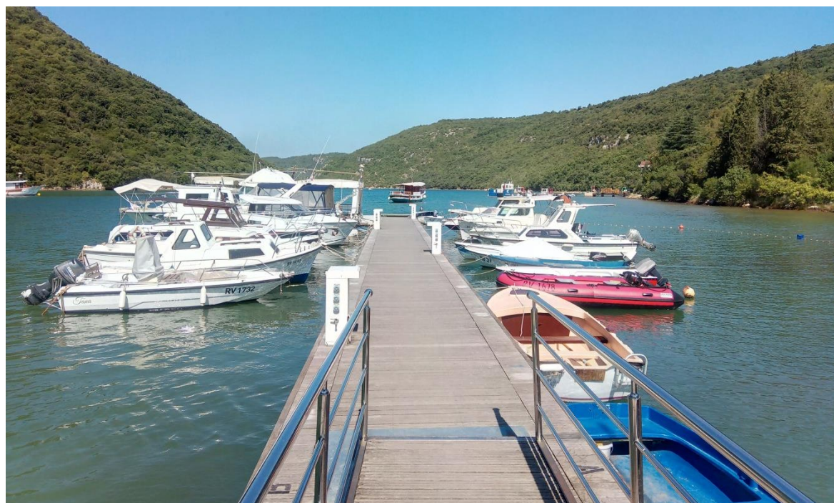
Figure 10: Marina at the Lim Channel – lower part.
