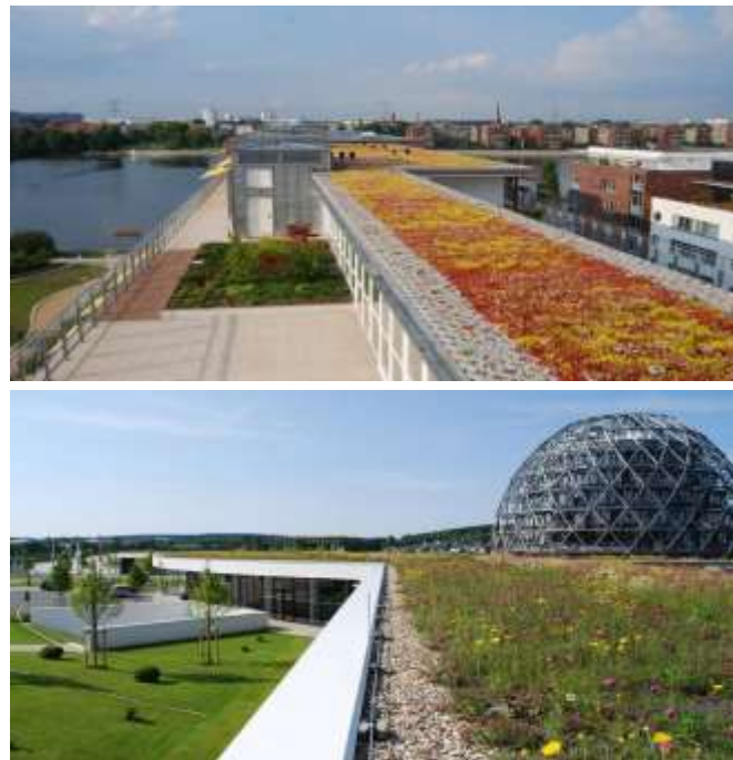
Figure 6: Examples of green roofs. Left: green roof with low biodiversity and a lower ecological value. Right: green roof with a high-level biodiversity and a high ecological value. Source: https://www.optigruen.com/
